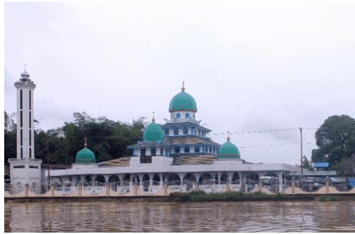
Picture 3. Sungai Banar Jami' Mosque Today
