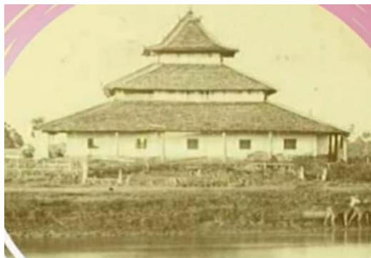
Picture 2. Sungai Banar Jami' Mosque Beginning of Construction
