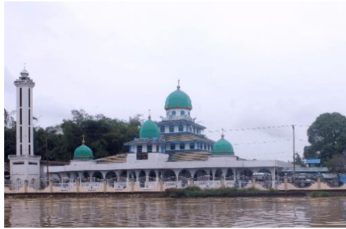
Picture 3. Sungai Banar Jami' Mosque Today
